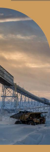
The Bloom Lake project is the first major iron ore project in eastern Canada since the 1970s. In 2018. Iron Ore Québec restarted the iron mine, located about 13 km north of Fermont. Québec. The mining company wanted to maximize profitability, so it upgraded its concentration plant and recovery circuit and commissioned the 3.5 km conveyor to reduce truck hauling.
